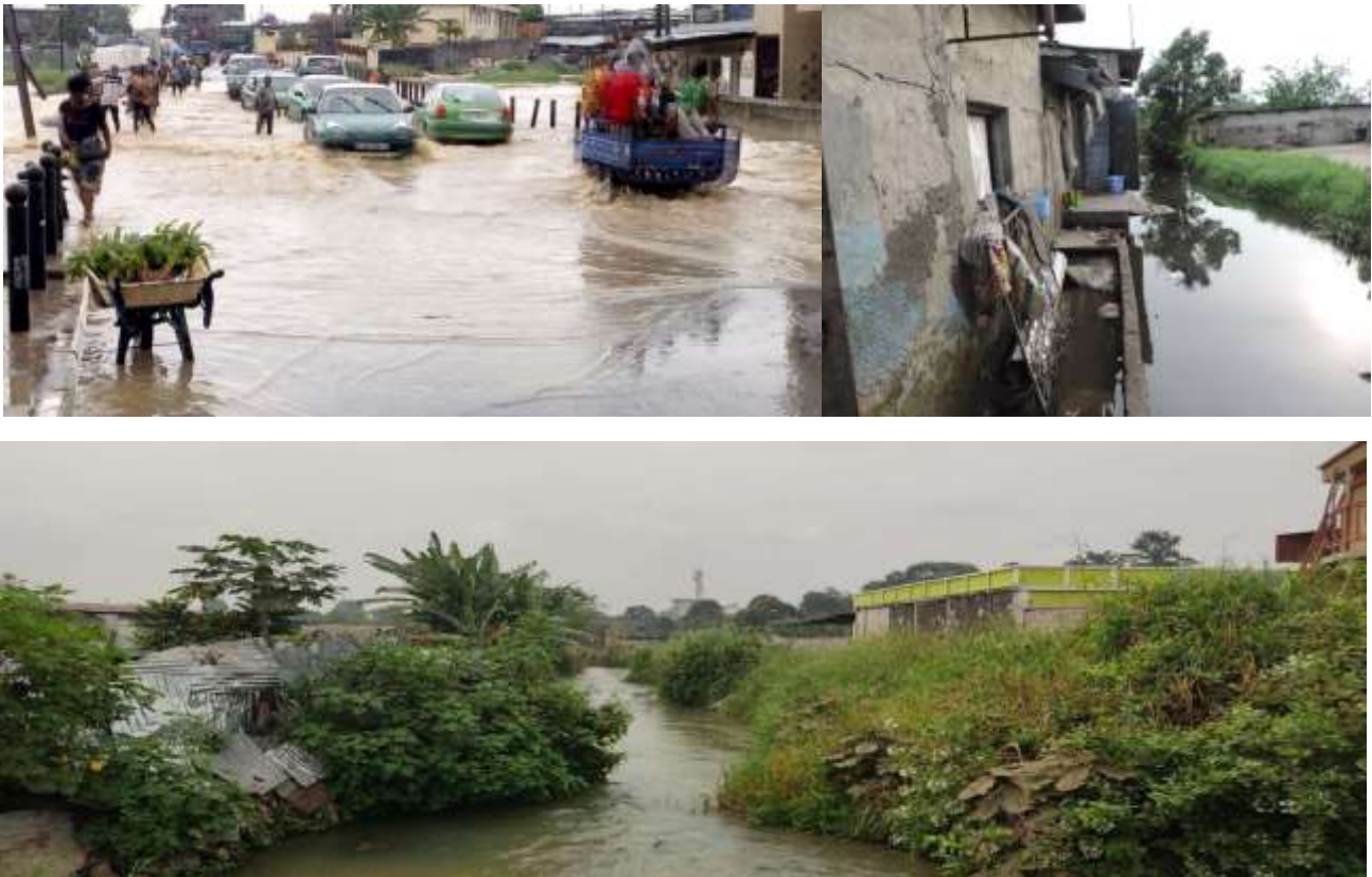
Photo 2: Flooding observed in the study area
