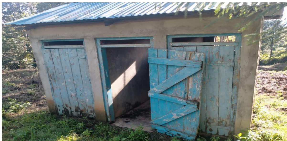
Figure 4: Teachers' latrines (own photo)
