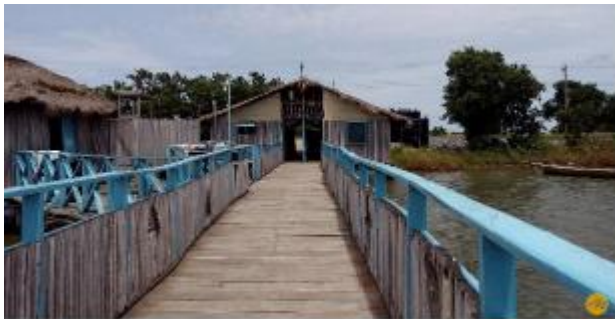
Figure 3: Wooden Platform (Pier)
