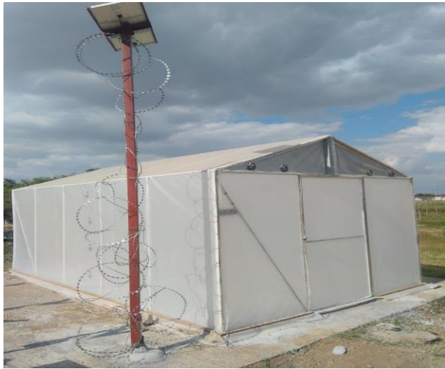
Figure 1. Greenhouse Solar Dryer
