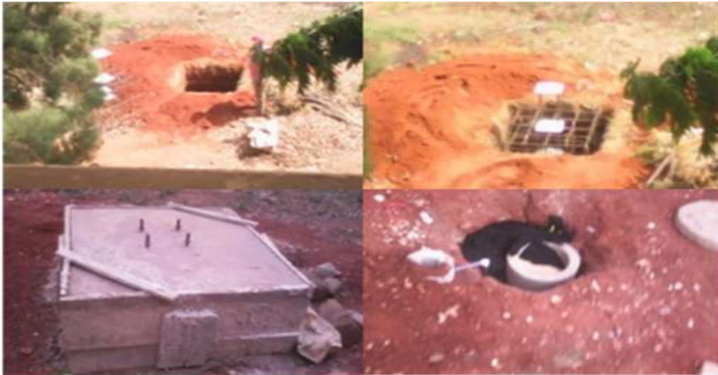
Fig. 3 Ground/concrete works for the VSAT installation
